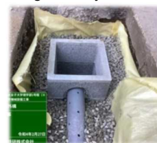
Rainwater infiltration pipe and rainwater infiltration trench
