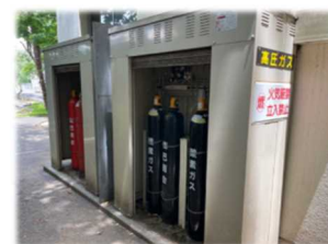
Cylinder Storage for Hydrogen and Oxygen
